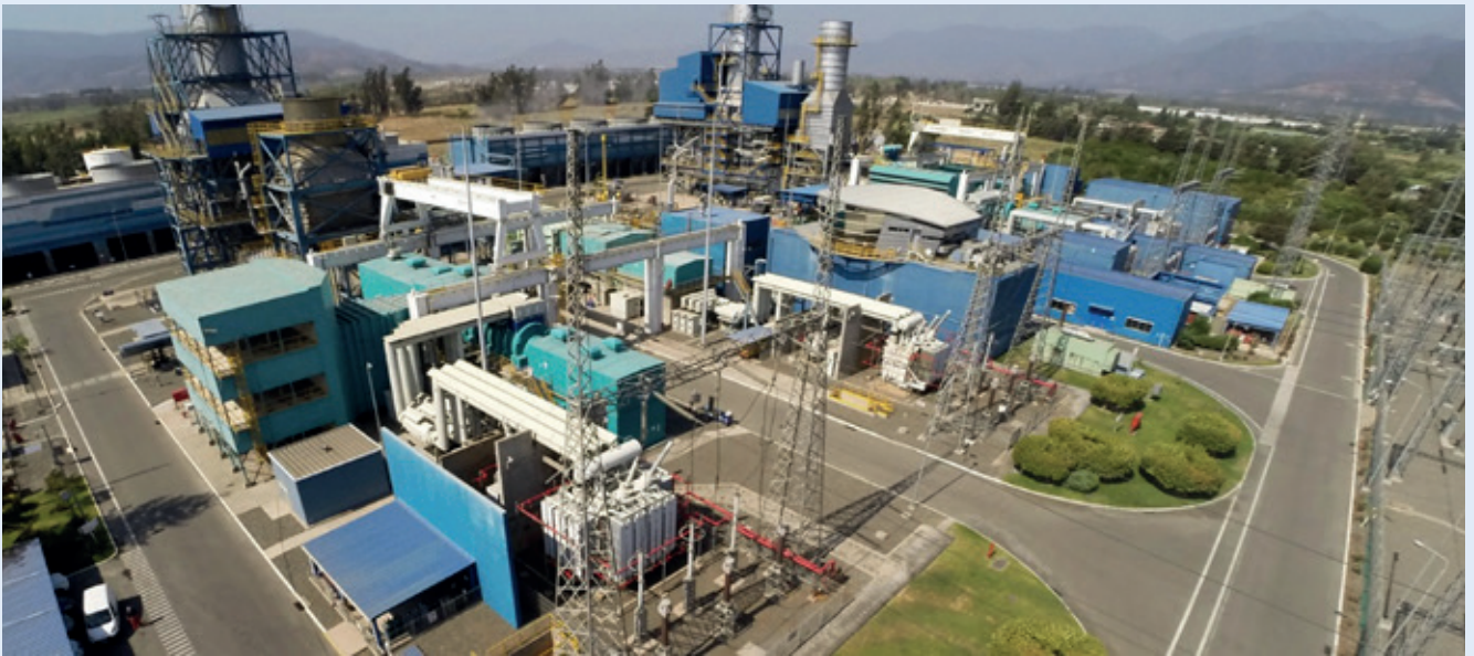
San Isidro power plant (Chile)
